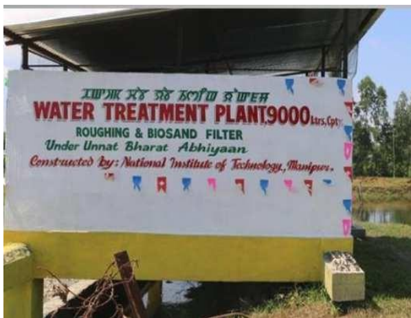
Constructed 9000 L Low Cost Water treatment Plant at Nambol (adopted village)
